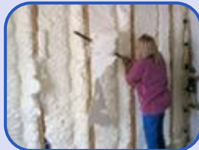
Icynene® foam insulation is made from the oil of the castor plant
