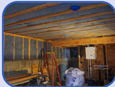
Denim insulation from recycled blue jeans
