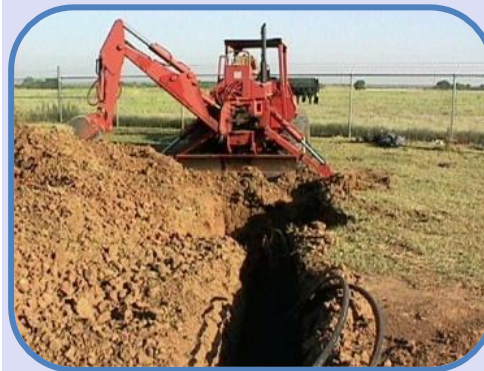
Excavation for underground loops
