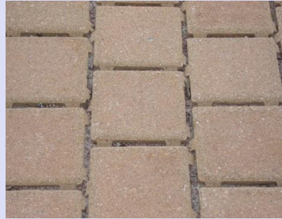
Interlocking permeable pavers
