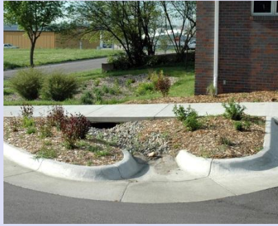
Sidewalk with curb cut
