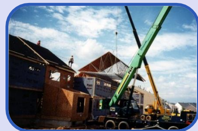
Prefab Roof Trusses
