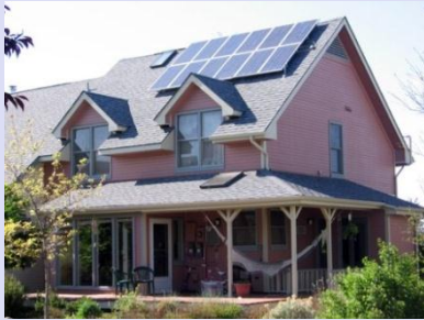
Solar panel retrofit
