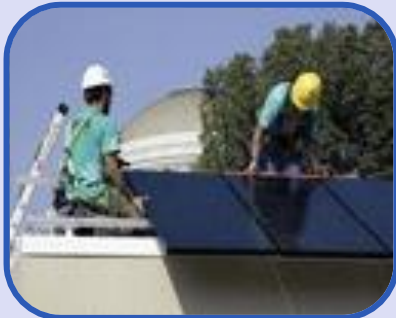
Solar panel roof installation
