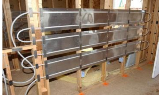
Radiant wall heater installation. Photo National Renewable Energy Lab, www.nrel.gov
