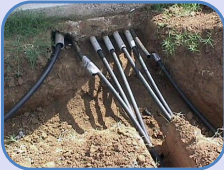
Geothermal system underground pipes
