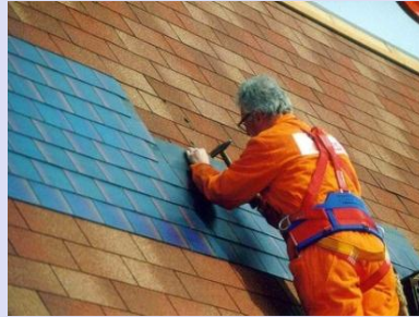
Solar shingle installation
