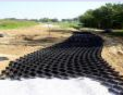
Pervious walking trail under constructions
