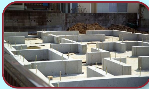
Foundations for a typical single-family home
